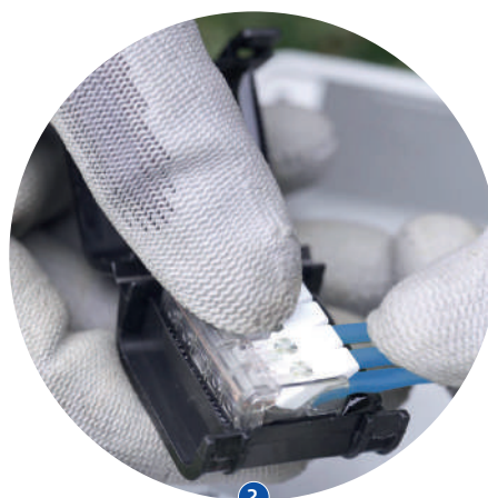
2 Posa del connettore cablato Laying of wired connector
